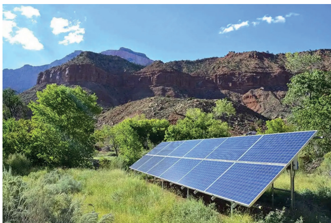
Figure 7. Solar panels installed on the ground [5]
