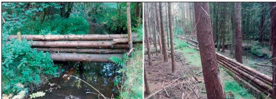
Figure 6. Woody debris dam (left side) and the flood storage bund (right side)
