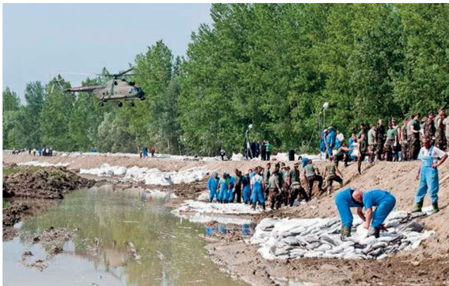
Figure 2. Soldiers and water management professionals are fixing the dike at Győrújfalu (Source: Krizsán Csaba, MTI)
