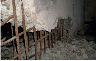
Figure 4: Reinforcement of structure Source: Photographed by the author
