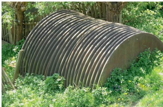
Figure 9: Corrugated sheet covering used for bunker interiors (valley block of Körösmező)
