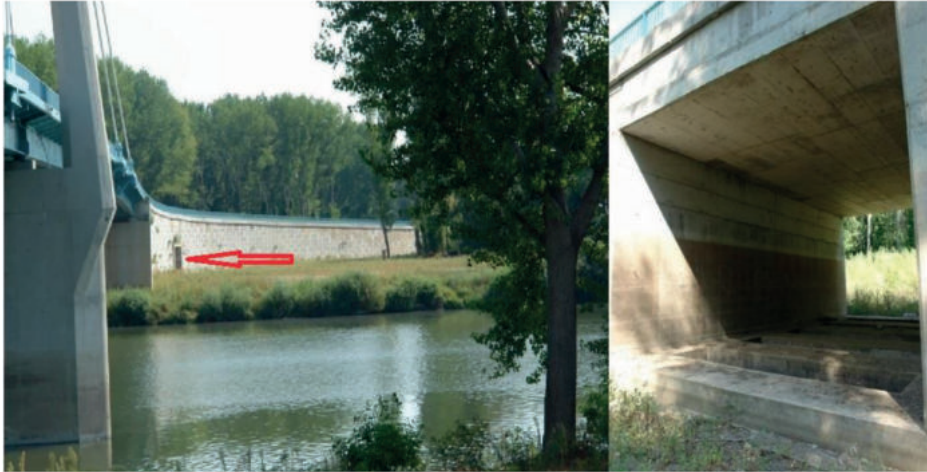
Picture 3. The picture of the openings on the Bridge of Ada
