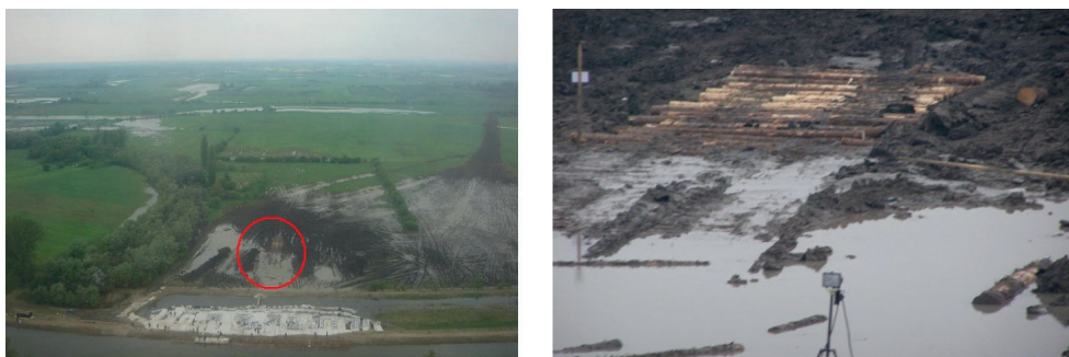
Figure 3. Flood protection road made of logs in an agricultural area near Csongrád in 2006.
