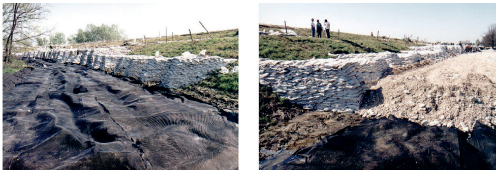
Figure 2. Construction of flood protection road of gravel at Tizsasüly in 2000.
