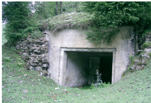
Figure 12: Anti-tank gun bunker near Oroszmokra
