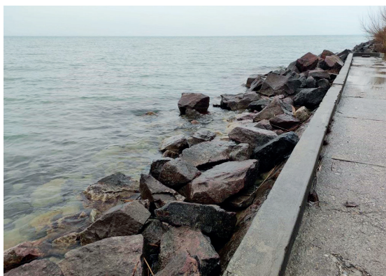
Figure 3. Protective embankment on the shore of the Lake Balaton
