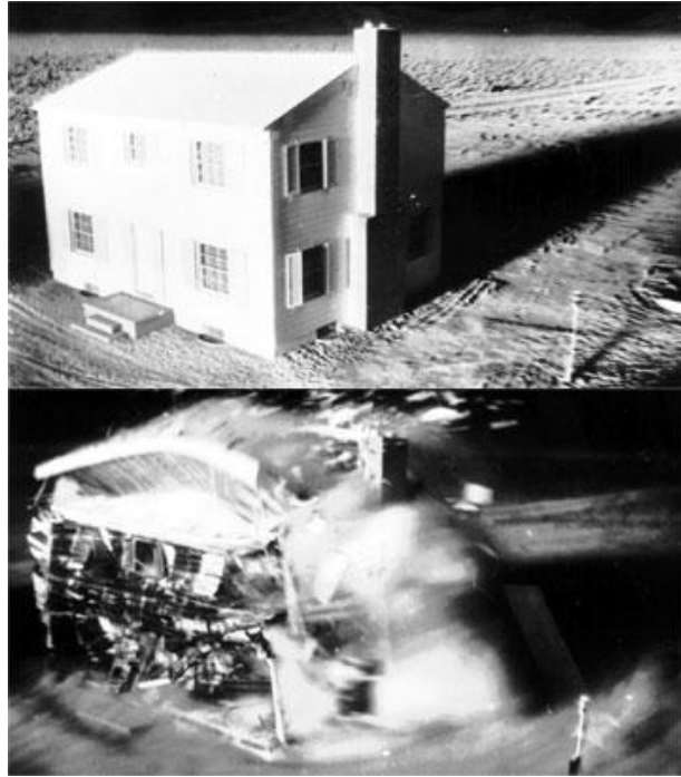
Fig. 4 Effects of the blast wave on a typical wood framed house [4]
