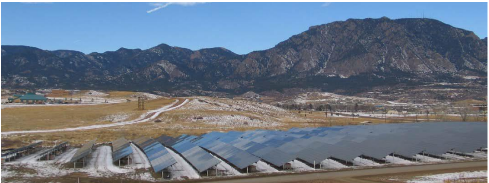
Figure 4: Fort Carson solar array. 11 (9)
