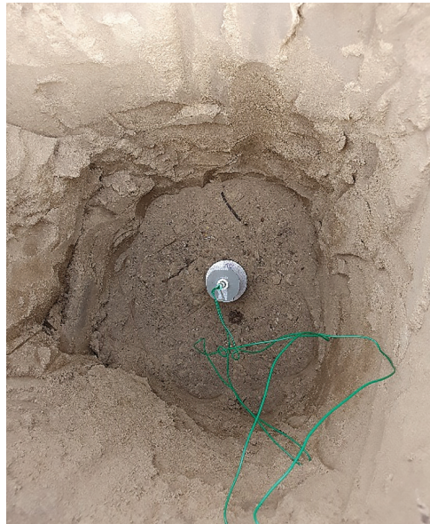
Figure 4: A charge placed in the blasting hole
