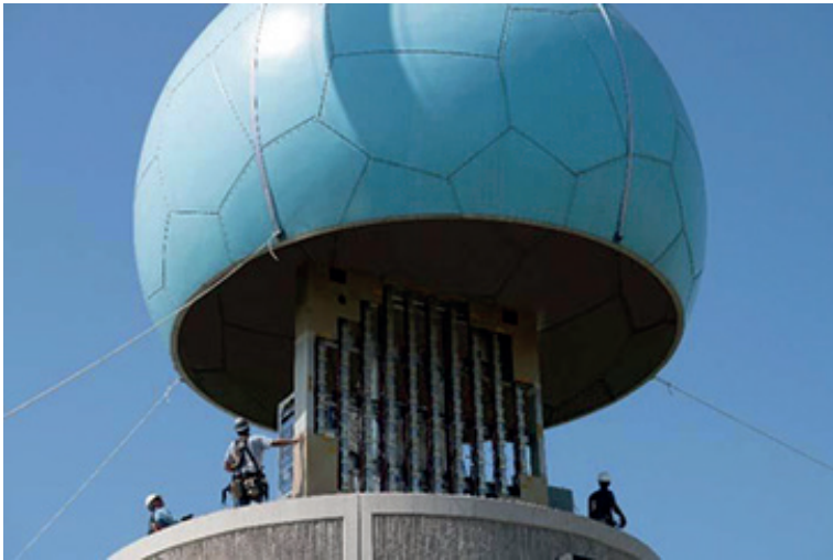
Figure 4 Installation of the NWRT RADOME in July 2018 [2]
