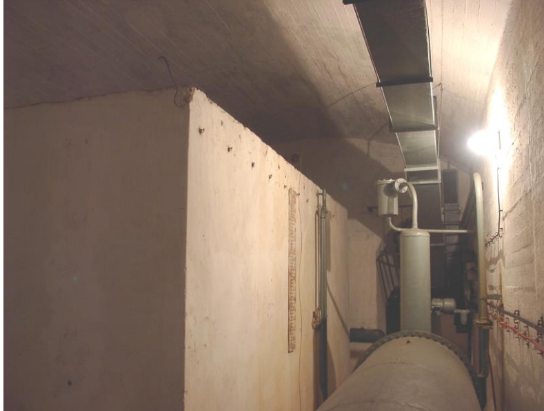
Figure 16: Reinforced concrete drinking water container in the Hospital in the Rock in Budapest 26
