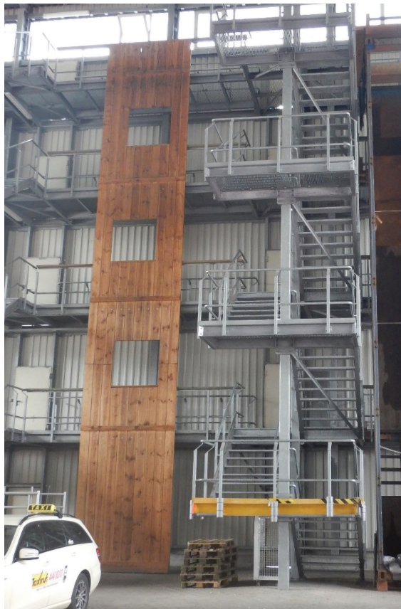
Picture 18: Multiple drill installations simulating tall buildings in a closed hall at the Firefighting Academy of Hamburg, Germany
